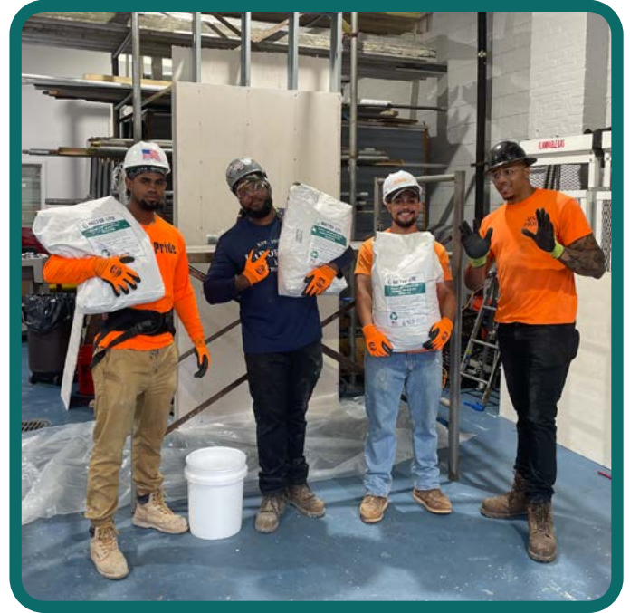
Pictured above: Belter Cem-Rock wall assembly behind workers
