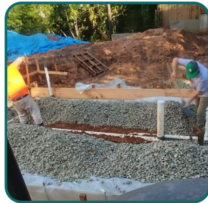
Pictured above: AERO Aggregates G15 used for sub slab compaction and insulation
